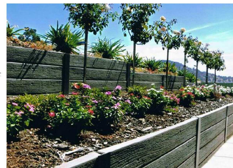
LANDSCAPED TERRACED RETAINING WALL EXAMPLES
